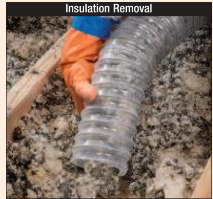
Insulation Removal
