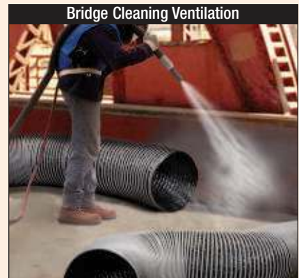
Bridge Cleaning Ventilation
